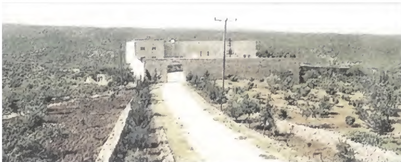
• A view from north side of the Monastery.
