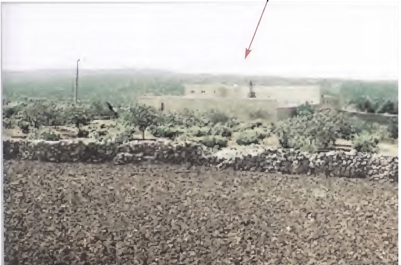
Two flattedbuilding at the west was built up by Priest Isho Atash is shown by the arrow.
